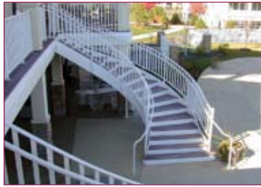
Custom Aluminum Staircase & Railings
